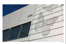
Lindab has developed a way of creating your own expression on facades. The customer chooses the motif to be shown, for example an image, a logo or text. Pattern perforated facade cassettes are used to create the motif on the facade, which can either be a small area or an entire wall section. The solution is called Lindab Art and allows architects and designers to give their building a distinct look. The possibilities are endless.
