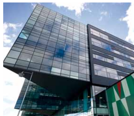
Lindab's air-tight duct systems and energy efficient chilled beams have helped to secure "Green Building" status for Lindholm Science Park in Gothenburg. "It is easy to work with Lindab. We receive tremendous help to find the best solution every time," says customer EU ventilation.
