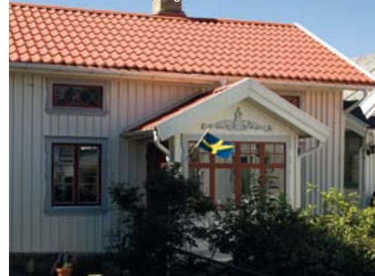
Residential house in Sweden with Rainline and Lindab tile effect roofing
