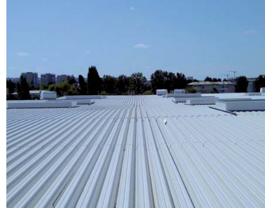
Roof solution for Baumax, Austria
