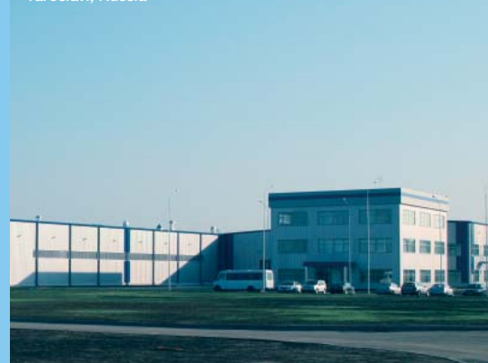
Lindab's newly opened plant in Yaroslavl, Russia
