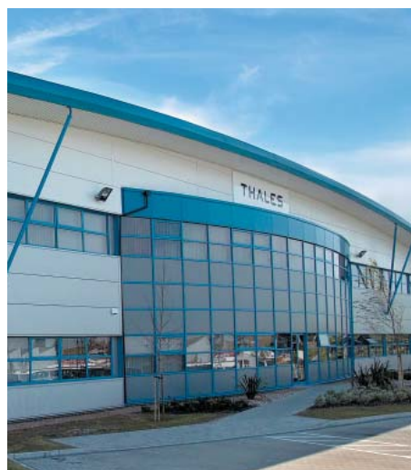
Pre-engineered steel construction in Hungary.
